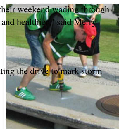
Volunteer installs environmental marker near a storm drain. Photo by
