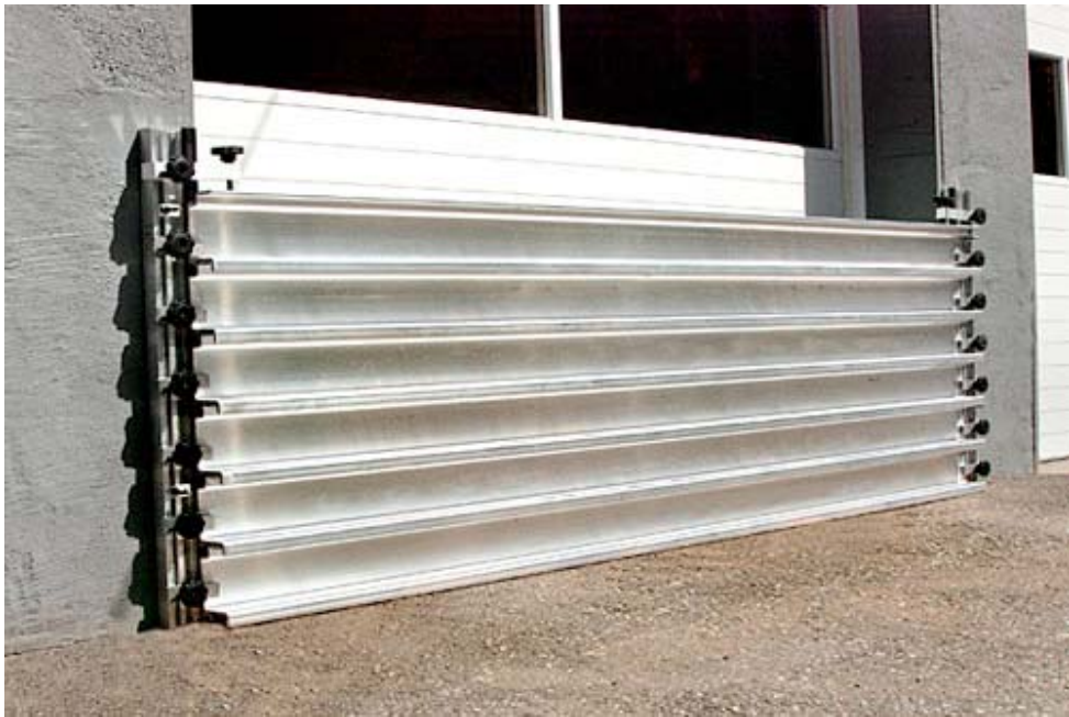
A series of interlocking, aircraft-grade aluminum planks will provide floodwater barricades at 16 door openings at Hilton and Scheman. Poured concrete walls that replace former metal or glass wall panels is another strategy the university will use. Photo provided.
