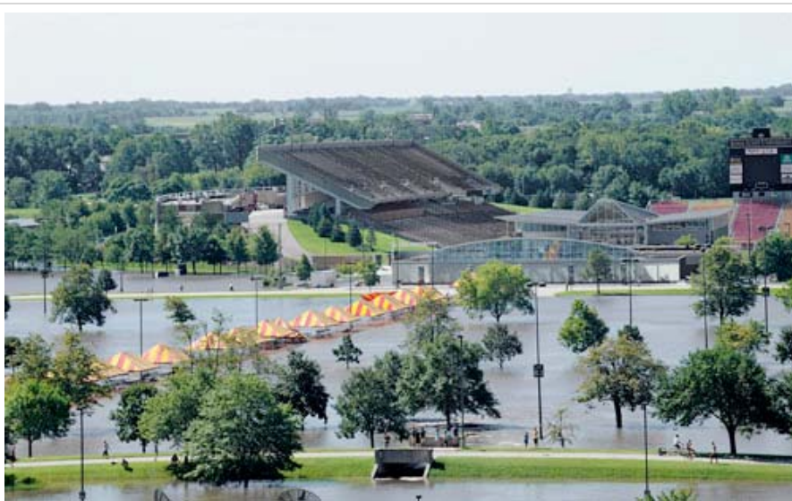
Flood waters inundated the Iowa State Center parking lots on the southeast side of campus the morning of Aug. 11. Photo by Bob Elbert.
