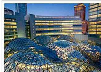
Atrium of the Zlote Tarasy office and entertainment complex in Warsaw, Poland. Nadia Anderson supervised the engineering design and construction for this portion of the complex. Submitted photo by Waagner-Biro Group.
