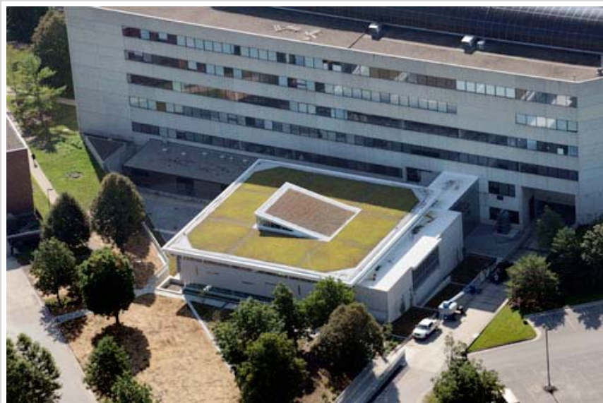
King Pavilion's green roof. Photos by Bob Elbert.
