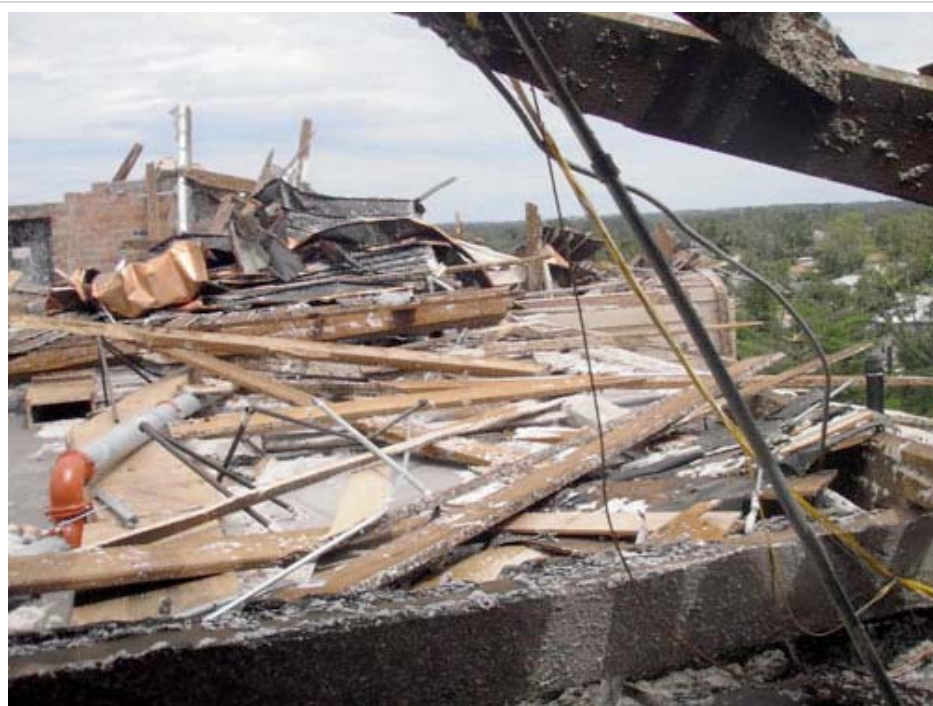
The Iowa Braille School's historic Old Main building sustained the heaviest damage from a July 11 storm. Nearly the entire roof and its support structure were swept away. Contributed photo.
