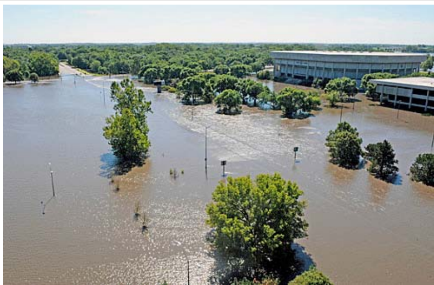
Floodwater at its peak the morning of Aug. 11, 2010, topped Lincoln Way, as viewed from the roof of Larch Residence Hall. Photo by Bob Elbert.
