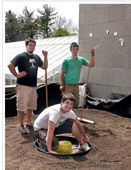
Members of the landscape and horticulture clubs helped install Horticulture Hall's green roof. Photo by Karina Antonetti.
