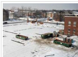
State Gym construction
